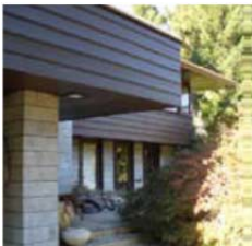
Cantilevered Upper Floors
