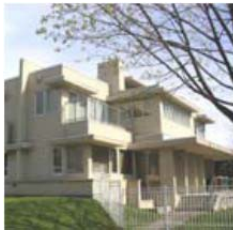
Horizontal Bands of windows
