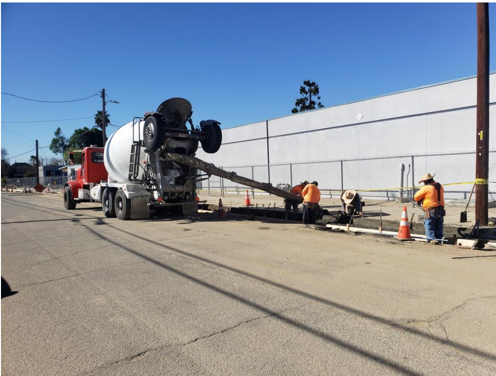
Placing new curb & gutter on Granada looking south to Ramona (Area 3)
