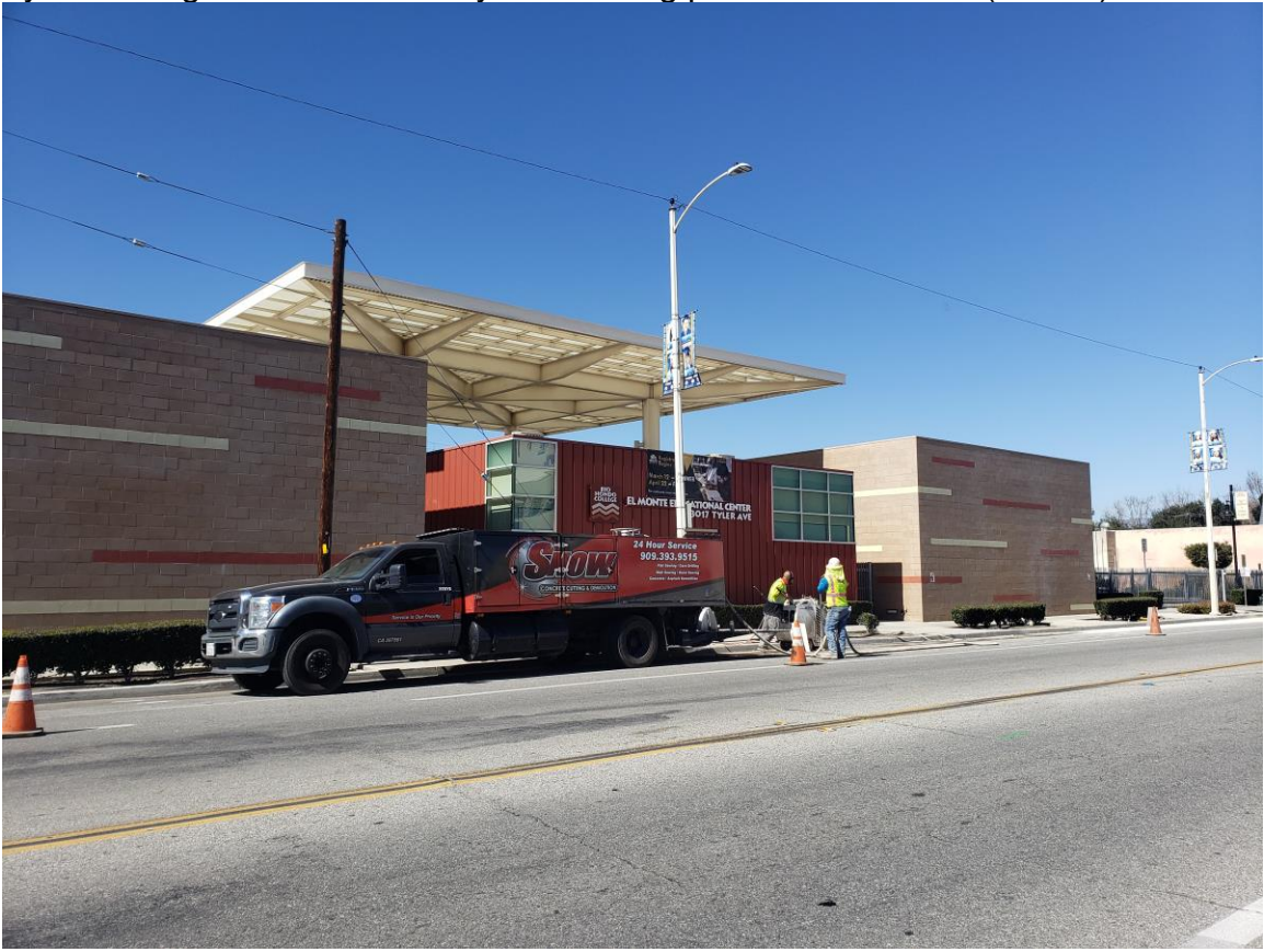
Tyler looking north from Garvey saw cutting prior to excavation (Area 1)
