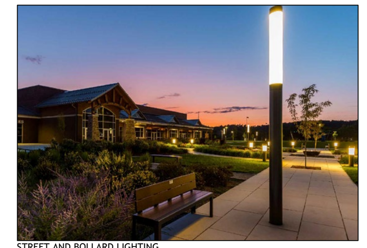
STREET AND BOLLARD LIGHTING
