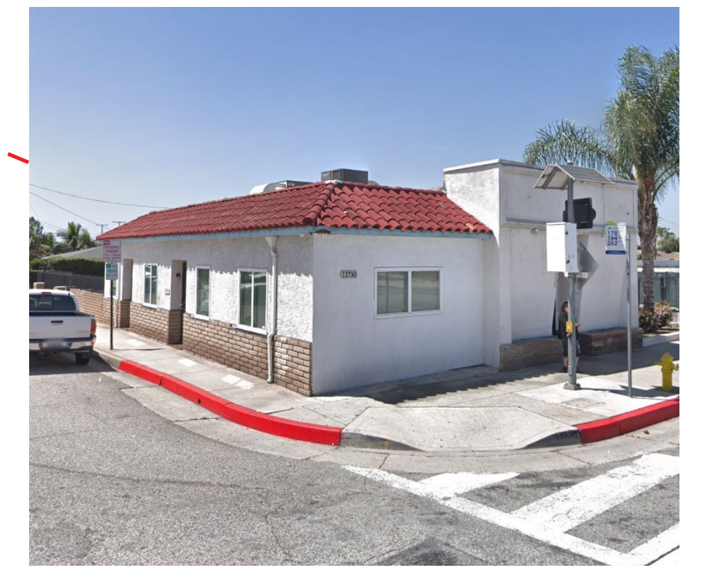
EXISTING 1-STORY OFFICE BUILDING TO BE DEMOLISHED - 1,875 S.F.
