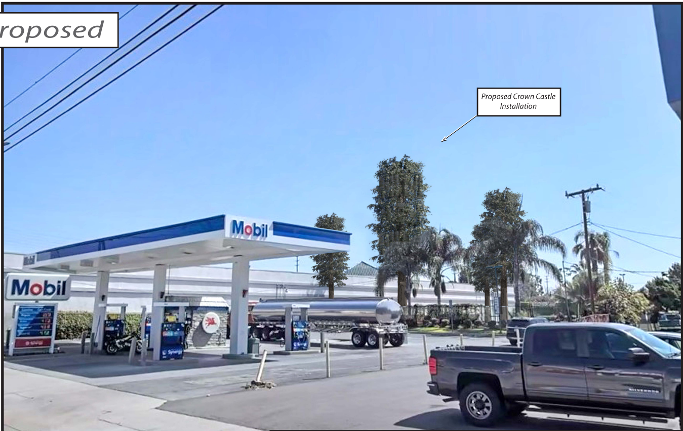
view from Peck Road looking northeast at site
